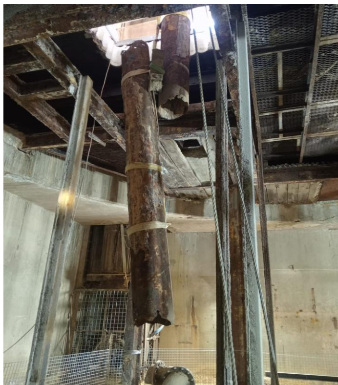
Photo 1: Hutchings Shaft redundant pipe removal.
