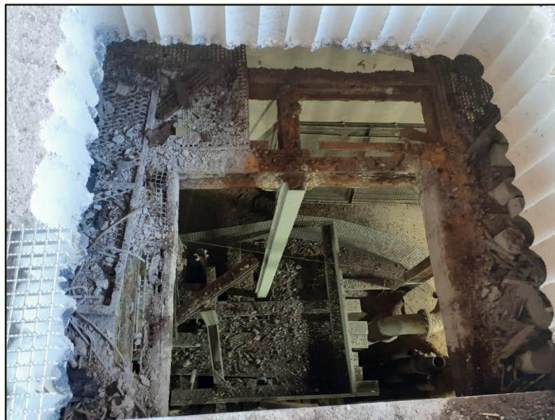
Photo 3: Hutchings Shaft Cement Slab Opened.
