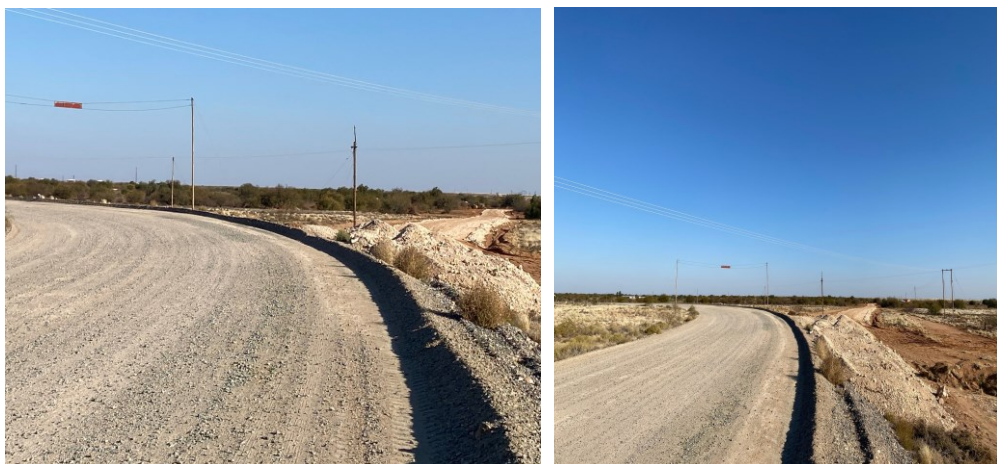
Photos: New Alkantpan road under construction.
