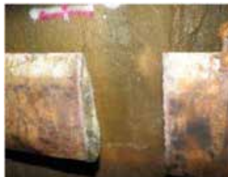
Location of removed section from underground bunton
