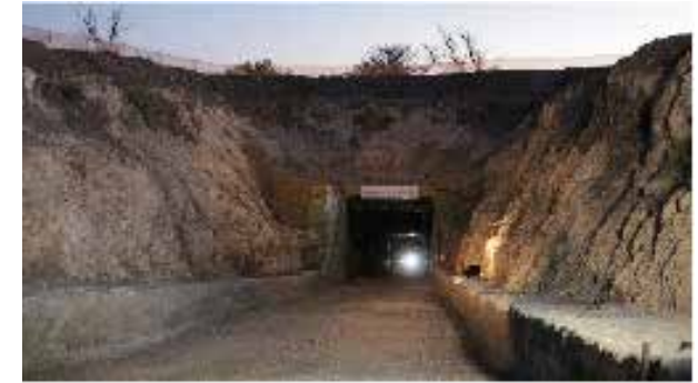
Surface portal access
