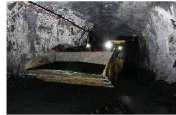
Existing underground haulage
