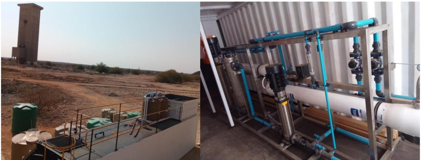
Figure 3: (LHS) Water treatment pilot plant mobilisation. (RHS) Commissioning the chemical treatment, filtration and reverse osmosis components of the pilot water treatment plant, setup to operate at 5m<sup>3</sup>/hr of feed water.
